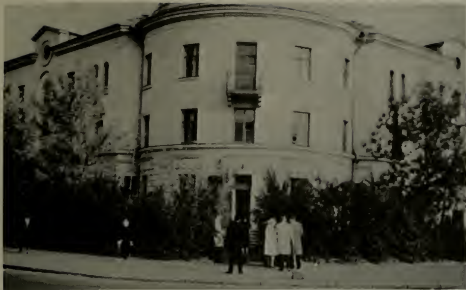
The workshop building at a Moscow NP Dispensary.
